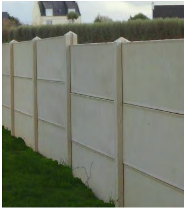
PLAQUES LISSES BETON MOULE
